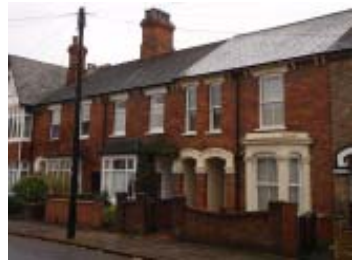
Original clay tile roofs and concrete tile replacement
