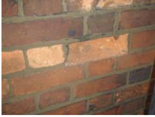
Examples of poor brick and stone pointing
