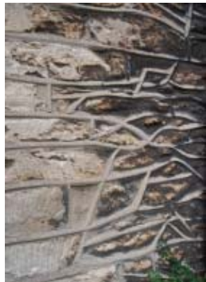
Inappropriate bucket handle joints and ribbon pointing
