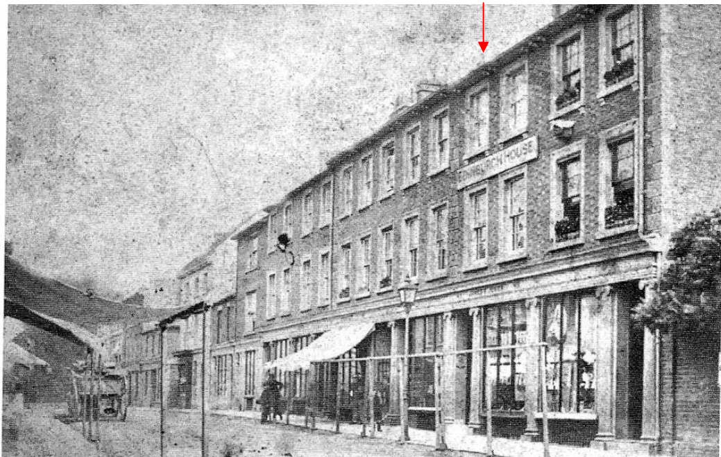
95 – 105 High Street in 1869. Note the structures to support the shop canopies. (Photograph source – BLARS)
