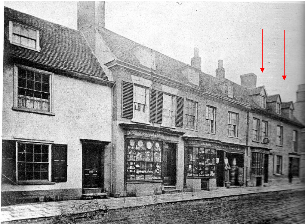
Nos. 86 – 88 (right) in 1870. No. 86 was occupied by Holmes & Co, fancy goods and tows and No. 86 by Malden's Bakery. (Source BLARS - original source Town Hall)
