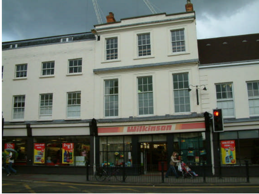
Central section of Wilkinson
