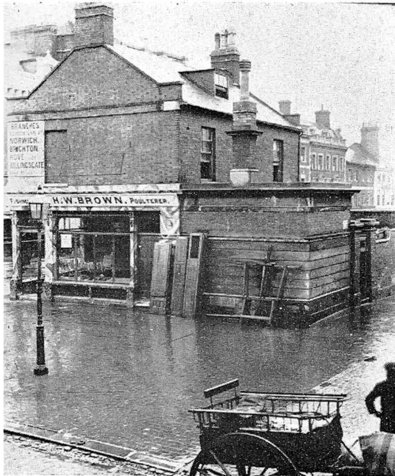
(No. 16) Brown's fishmonger and poulterer. Photographed just prior to demolition in 1895. (Photograph source – BLARS)
