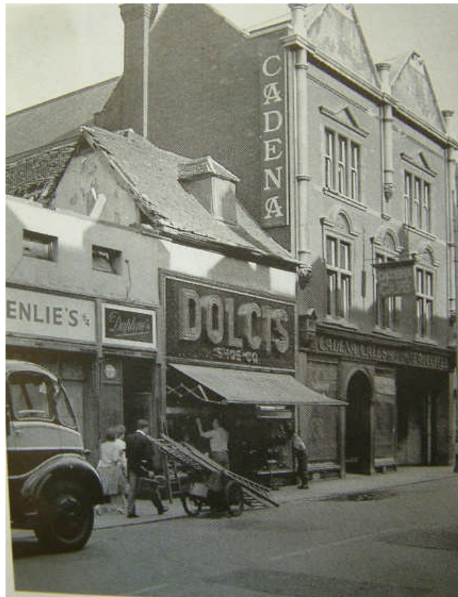
No. 66 in 1960, sporting a large 'Dolcis' sign . Demolition work appears to be in progress at No. 64. (Photograph source – 'Bedford', Richard Wildman)
