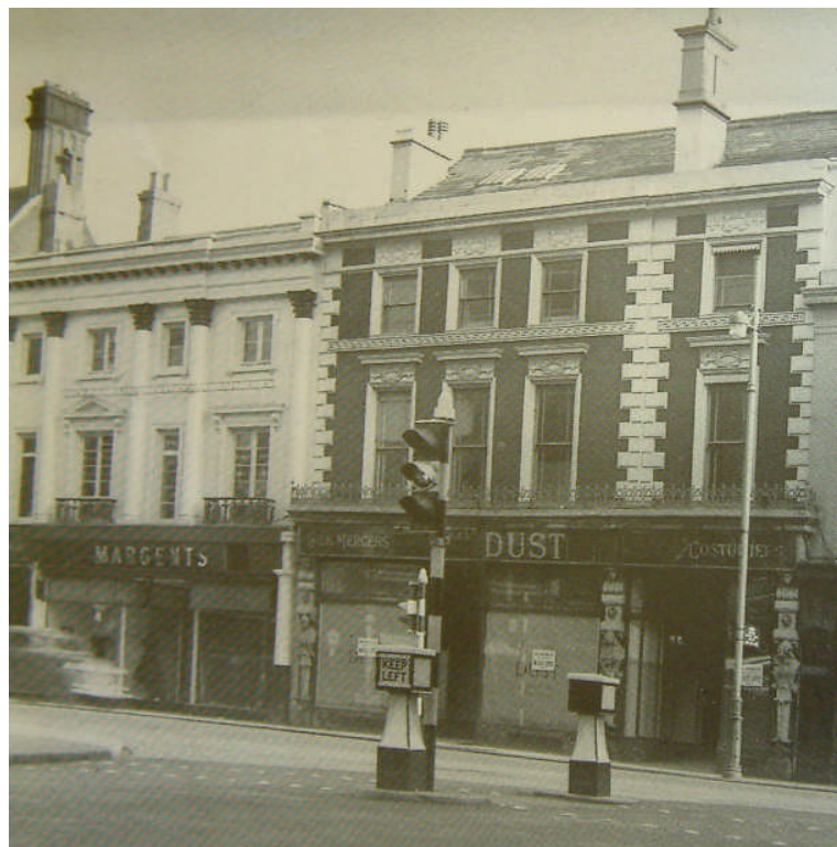
No. 75 c1957, just prior to demolition. (Source 'Bedford', Richard Wildman)
