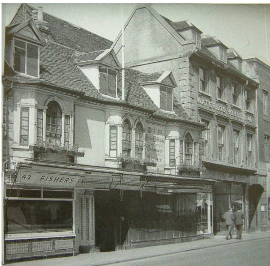
Nos. 42, 44 and 46 in 1957, prior to demolition in 1963. (From 'Bedford', Richard Wildman)
