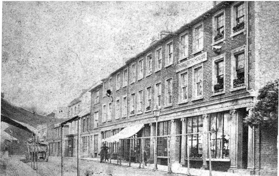
95 – 105 High Street in 1869. Note the structures to support the shop canopies. (Photograph source – BLARS)
