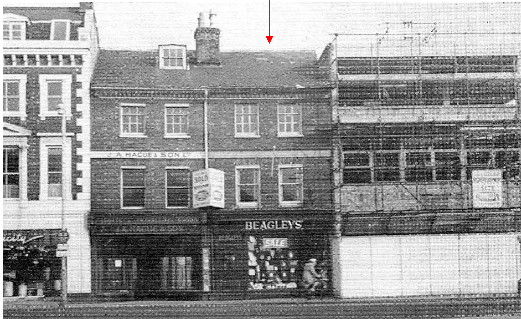
The first section of Swan Court is being constructed following the demolition of Murkett Bros (formerly George Hotel), right, in 1959. Nos. 5 and 7 are still standing in this photograph but were demolished shortly after to become part of Swan Court.
