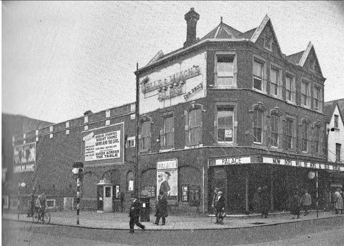
1935 after Inn converted into Palace Cinema. (Photograph source – BLARS, Gearey negatives)
