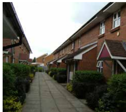
Raglan flats within the project
