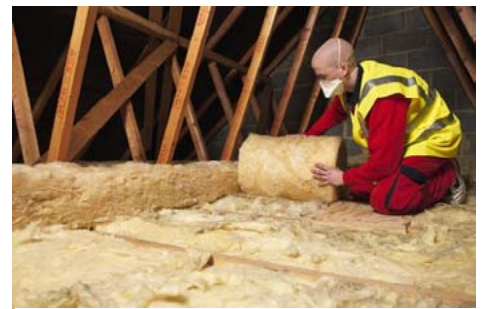
Loft insulation being Installed in a Loft
