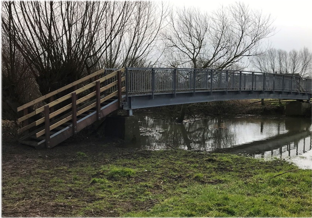
Back Channel Bridge
